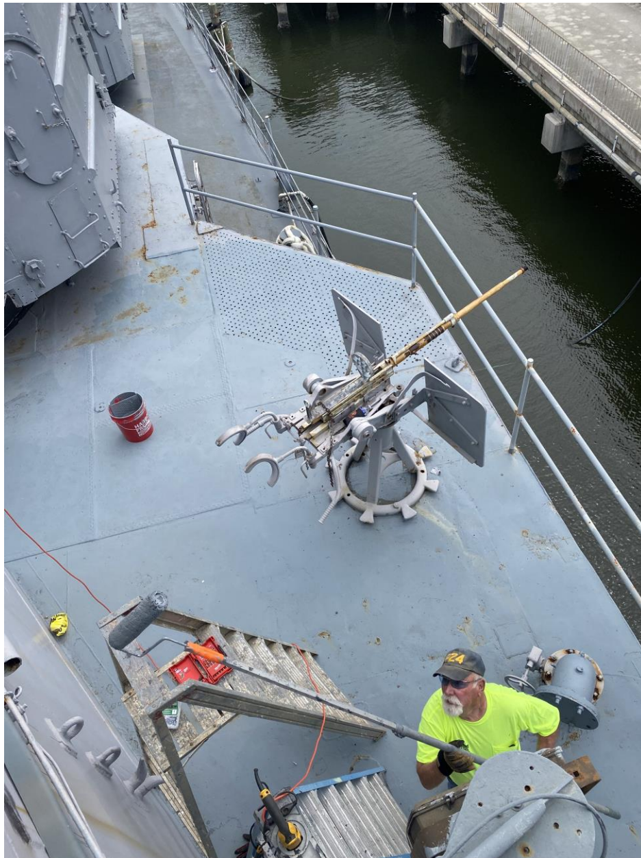
Tom Aust Painting Bulkhead on 01 Level
