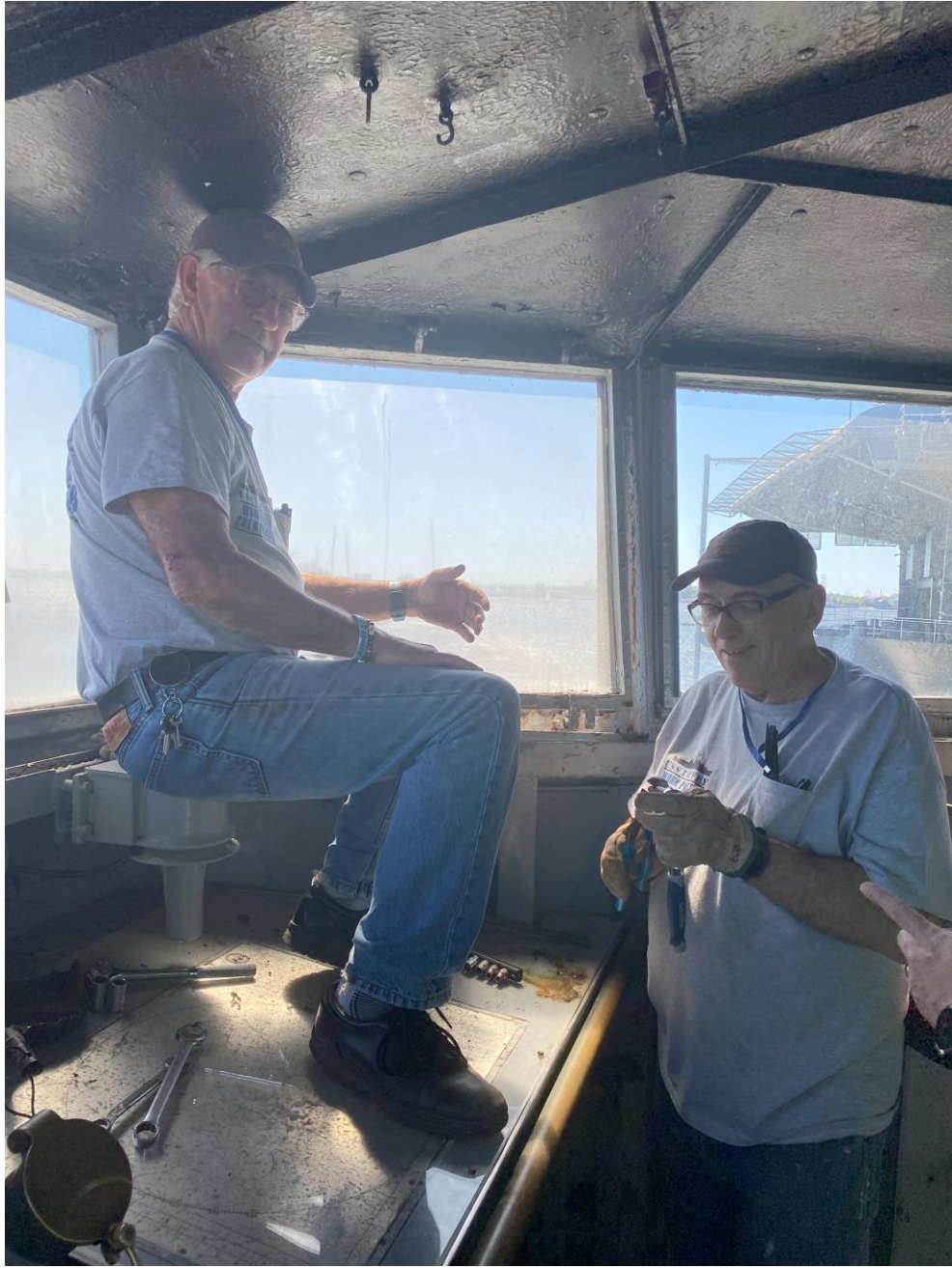
Harry Stoner and Ernie Doyle Repairing Leak on Bridge
