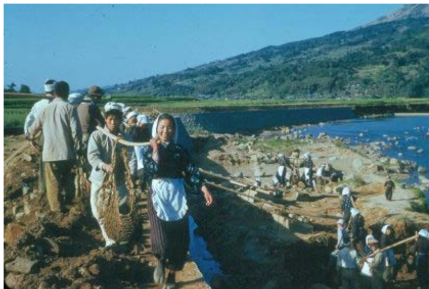
Sasebo, Japan. April 27, 1952. Karatsu women working on stone wall.
