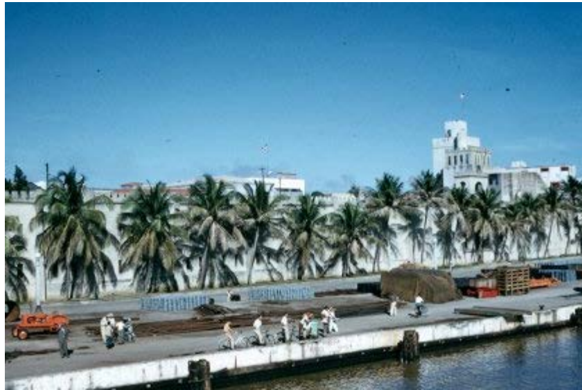
Ciudad Trujillo. Walls around city. NVD Docks - and top is Army fort January 31, 1953
