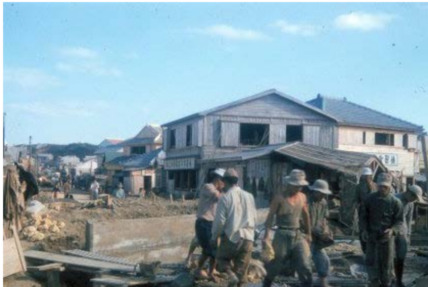
Naha, Okinawa. 5 April 1952 Laborers building a bridge
