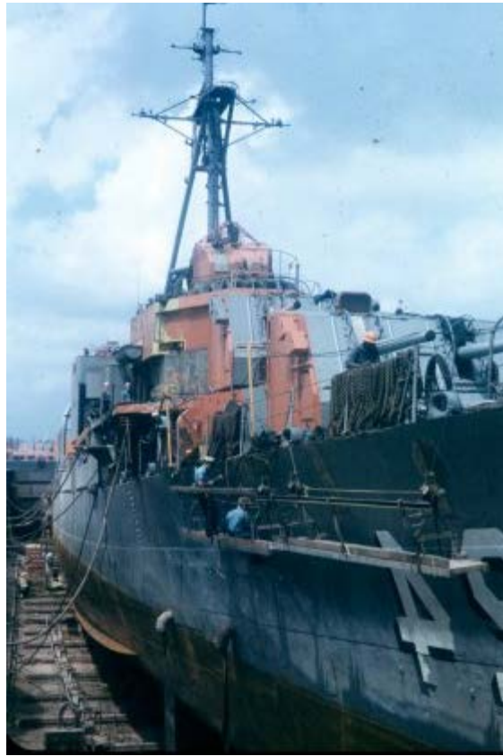
Portsmouth Yard. June, 1951 The Laffey being rebuilt with a tripod mast.
