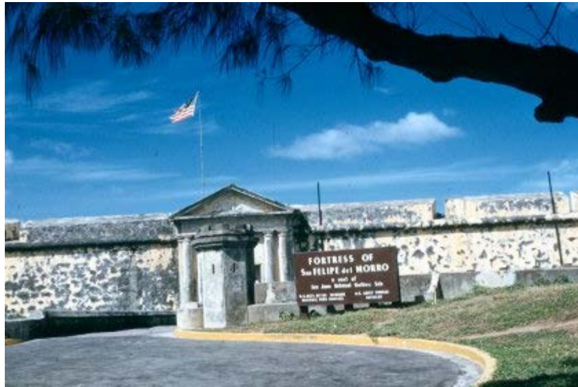
Entrance to golf course in moat of Fort El Morro January 25, 1953
