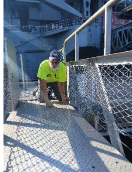
Marc Jacobs repairing netting on the gangway
